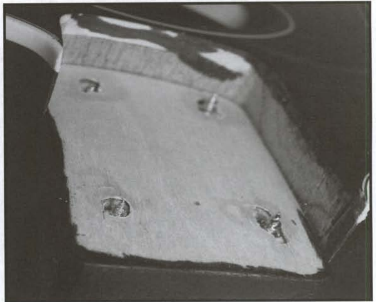
FIGURE 4.19 If the shim doesn't fully cover the pocket, it can result in tone loss and a warped neck. (Photo by John LeVan)
